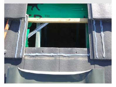
3- Fit Throat, Level, then tie down with 3 Straps to timber battens.4- Mount the 500mm Twista Rotary Head onto the throat to finish.
